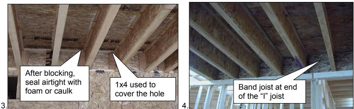
Pictures four and five show the use of a band-joist or ribbon closing the end of the "I" joist. If 2x8's or 10s are used as floor joists, the same dimension lumber and a band-joist of Oriented Strand Board or Plywood can be used to block them.
