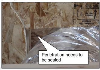
Picture 4 shows where the duct in picture 3 is penetrating the dropped ceiling cap. All penetrations should be sealed with foam, caulk or mastic.
