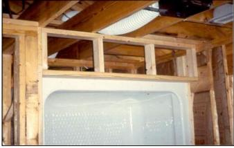
As shown in pictures three, five and six, it is best to cap all dropped ceilings during the framing stage with OSB, plywood, sheetrock or Thermo-ply. Insulation can be easily run across the framer-installed cap. This method assures a tighter house and insulation that performs to its capability.
