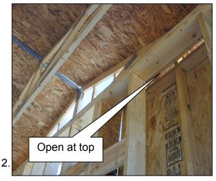
The easiest way to ensure this wall will not contribute to air leakage and insulation failure is to place rigid sheathing such as oriented strand board (OSB), plywood, sheetrock or Thermoply<sup>TM</sup> on the back side of the interior wall as shown in pictures 3, 4, and 5.
