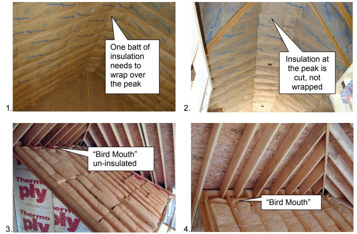
Pictures three, five and six also show that the insulation needs to be snuggly fitted at each intersection of insulation. These small voids add up to a large reduction in effective R-Value.
