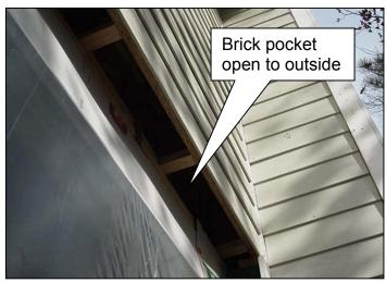
Picture three shows the interior side of the brick pocket. Insulation will not stop airflow. Picture four shows the underside of the brick pocket (exterior) that has been correctly sheathed and sealed.
